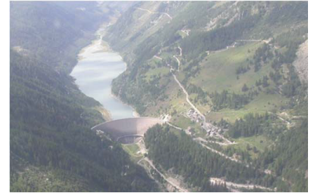
Open Theme Presentation: Rehabilitation of Beaugard Dam (Presented by RSE SpA)
